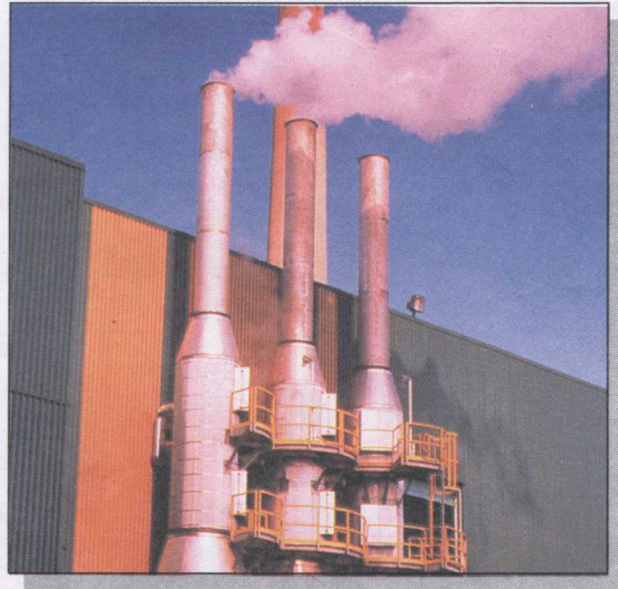
Steam venting from HBM&S zinc plant, Flin Flon
